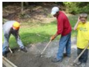
Arrowmen at work on an irrigation system
